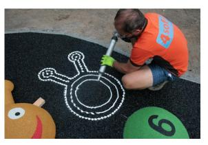
Spread one or two component glue evenly directly on SBR - TAKE CARE ABOUT UPPER SIDE OF COMPONENT TO AVOID STAIN OF GLUE ON IT!
