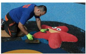
Apply the thick binder on outside edges of 3D component to avoid edge separation from the rest of the EPDM on the top layer. TAKE CARE ABOUT UPPER SIDE OF COMPONENT TO AVOID STAIN OF YELLOWING BINDER ON IT!
